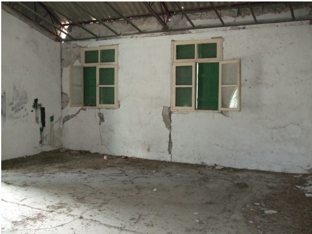
Figure 3: Aksylou/Aksu Mosque interior – note the old green paint.
